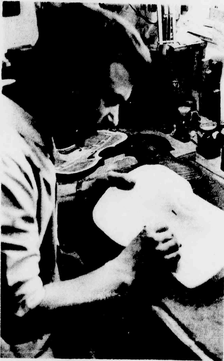
METICULOUS — Rene Morel, world famed stringed instrument repairman, works on the restoration of a rare violin.
